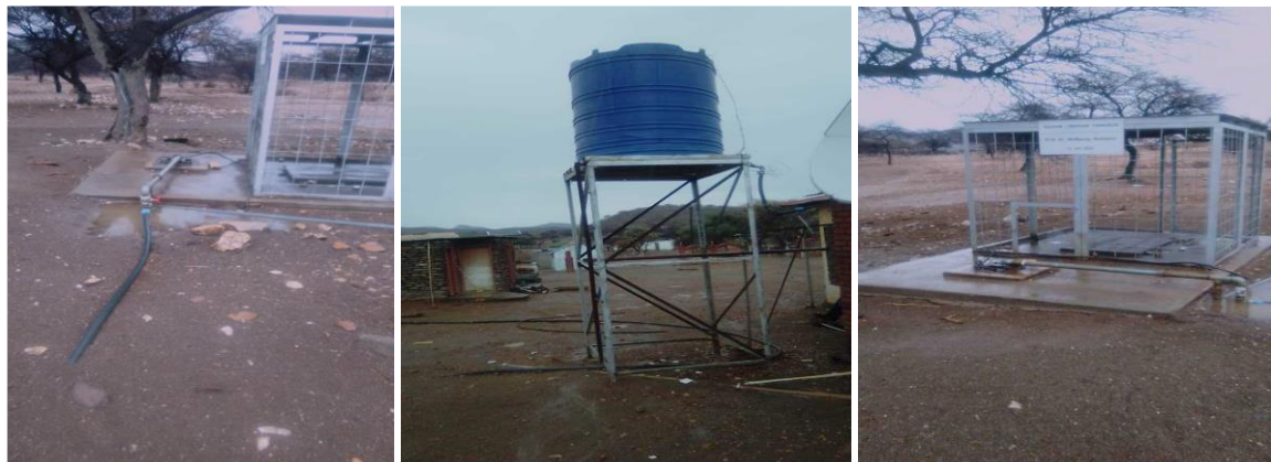
Figure 2. Pictures of some borehole water sampling sites.
